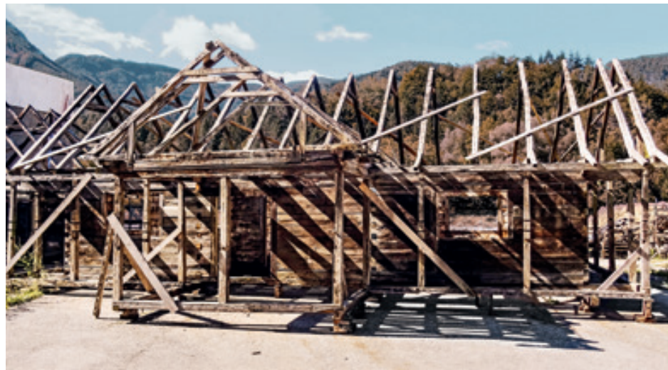
Altholz-Gerippe einer Scheune. / Old wooden frame of a barn.
